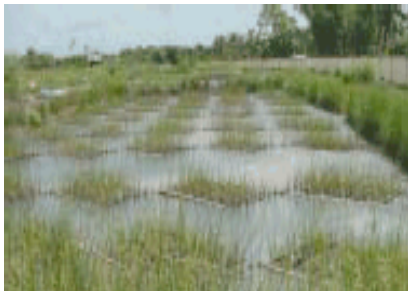
Polishing of wastewater effluent in China
